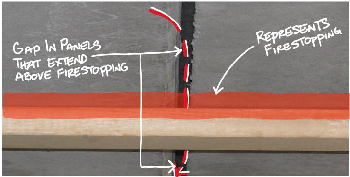
We cannot just seal the joint at the wall...this will not stop the passage above the firestopping.
