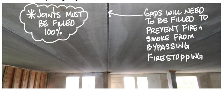
The gaps need to be treated, 100% of the length of the panel
